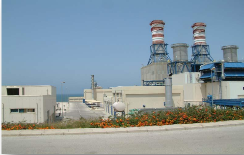
Beddawi Power Plant
